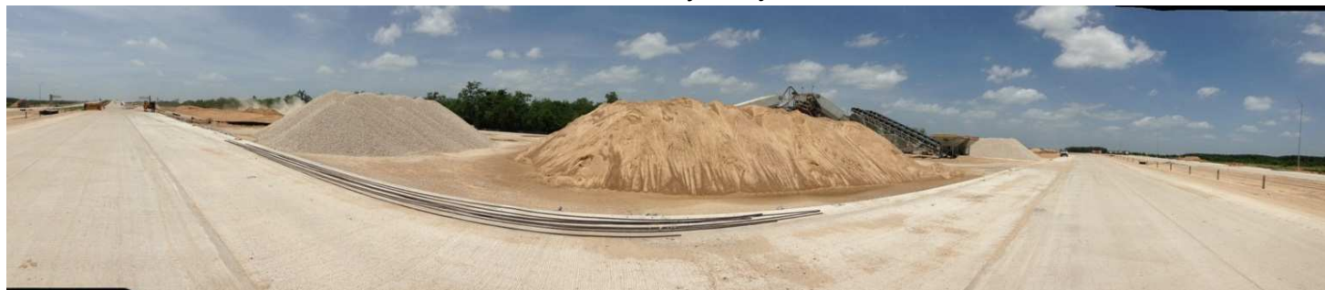
SH 99-Grand Parkway Project, Houston
